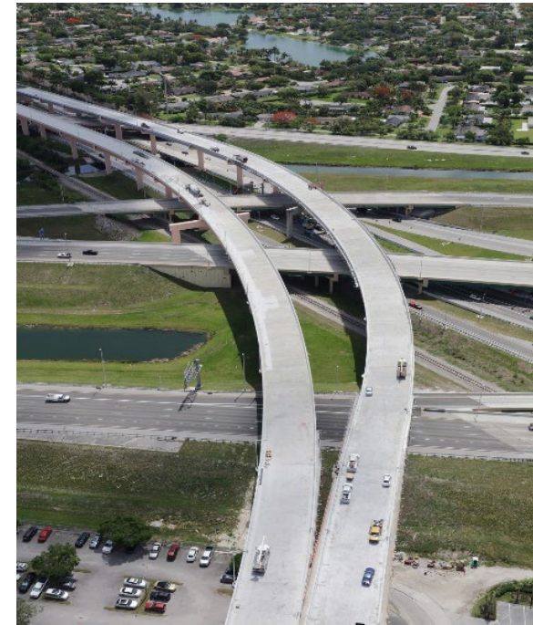
SR 874 Northbound/Southbound Connector Bridges to SR 874
